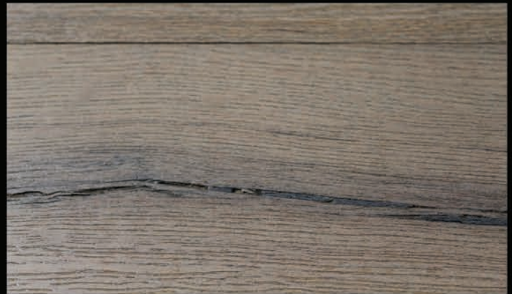
NAIL HOLES, SURFACE CHECKS
